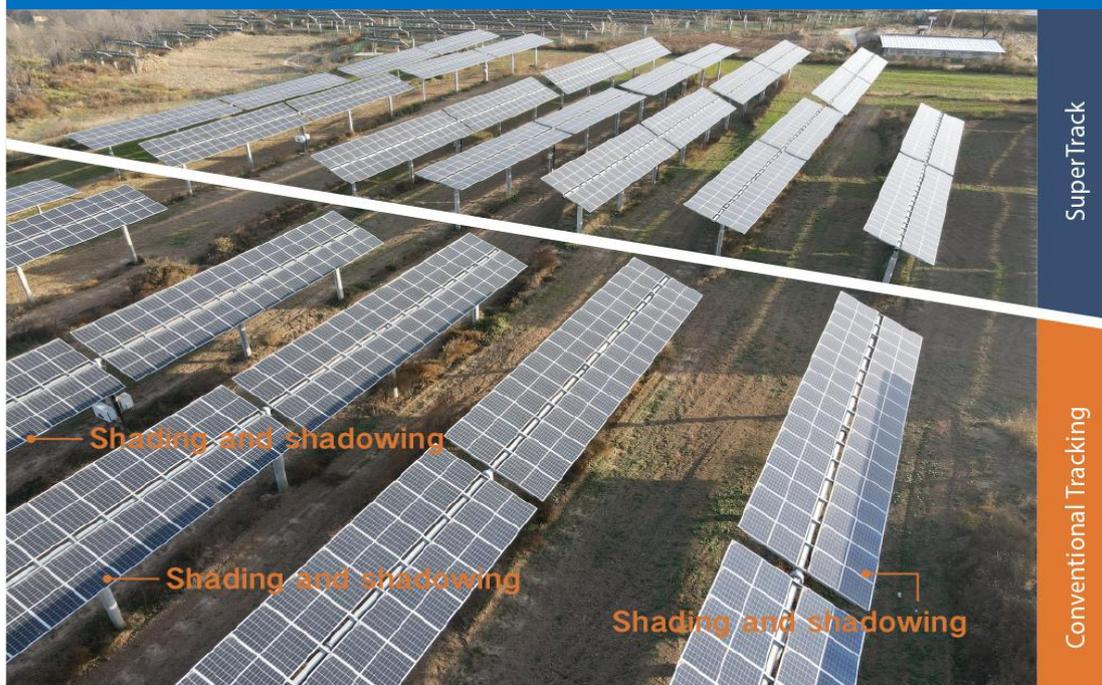
As shown in the figure 21, i.e. live photos of the test project in Tongchuan on sunny days at the stage of backtracking, shadow shade and light leakage can be found due to terrain difference in conventional tracking array. Therefore, SuperTrack array will optimize different backtracking angles for each row of arrays according to terrain conditions, reduce light leakage as much as possible while avoiding shading, and enhance power generation at the stage of backtracking.
