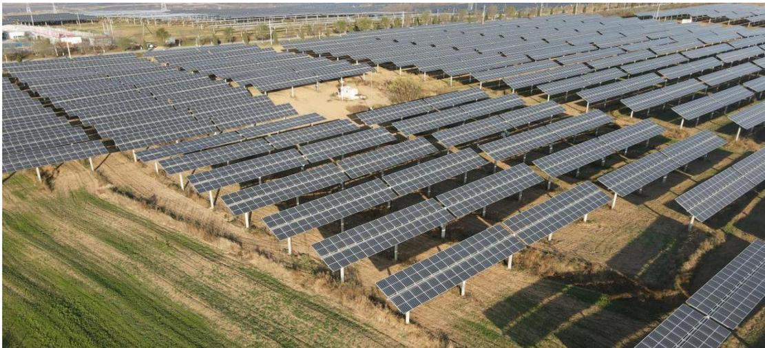
The power station is located in Yijun County, Tongchuan City, Shaanxi Province, China. It adopts bifacial module + horizontal single axis tracker system and selects megawatt-level photovoltaic arrays with similar terrain for verification. Specific project information is shown in the table 3:
