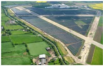
multicrystalline modules were installed in just three months, and the array was connected to the grid in March 2013, rendering the project eligible for full support under the Renewables Obligation Certificates (ROC) scheme, qualifying for 2ROCs. The output is around 30,650MWh, which is enough to power 8,000 households.
